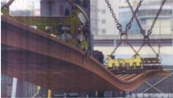
This type of object will tend to curl as the unsupported length increases. The lateral curvature moves the C of G to the side; this causes the object to tip and increases the curvature. This action can be very violent and cause personnel injury.
